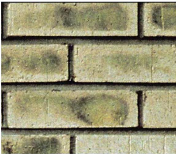
Bricks that are prone to vanadium staining often give an early warning signal after they become wet and have been allowed to dry out. Fresh brickwork that exhibits early vanadium staining should be brushed with a bristle brush and hosed down. If this approach fails, only then should alternative chemical treatment be tried.
