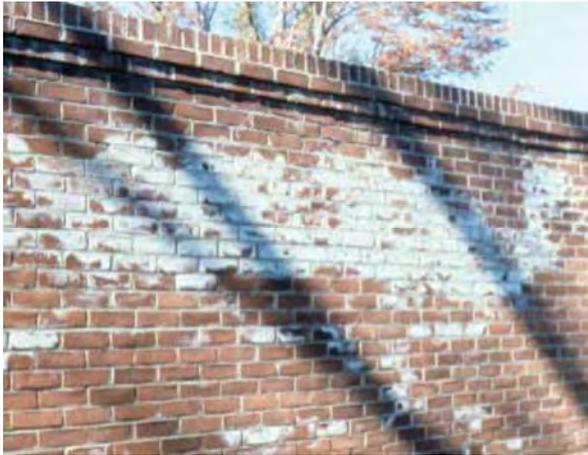
**Figure10.2: Wall with Efflorescence**
