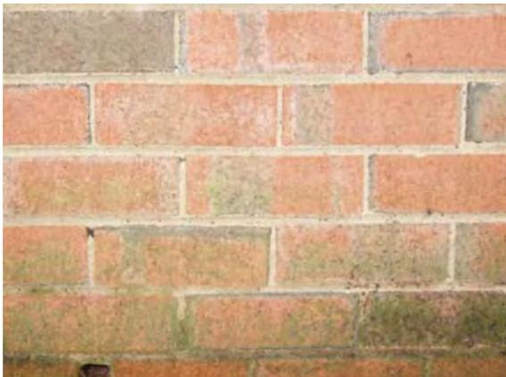
Micro-organic growths such as fungi, moulds, lichens and mosses on brickwork often cause unwanted dark stains or smears on portions of buildings and garden walls.
