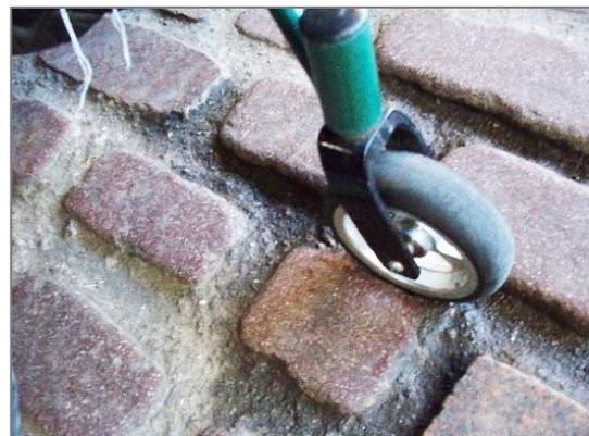
A frequent criticism of segmental pavements is that they have too many joints, which result in more vibrations to wheelchair users. However, vibration measurements conclude that the narrow joints in segmental pavements result in less severe vibrations than control joints in concrete slabs.
